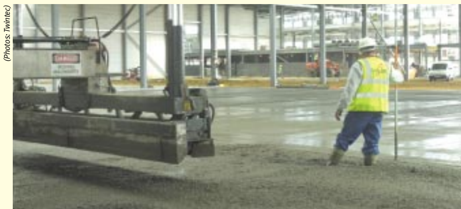
The concrete was a C40 mix incorporating superplasticiser, 50kg/m 3 of steel fibres and had a water/cement ratio of 0.5.
