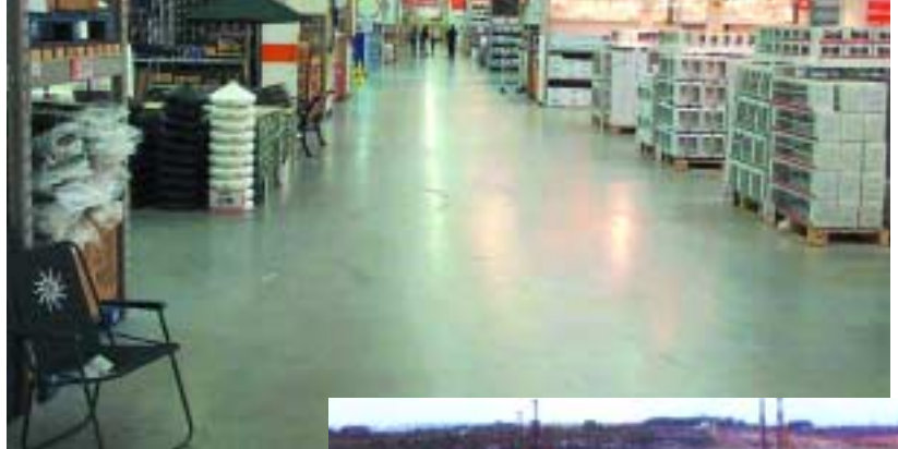
ABOVE: Figure 1: A finished steel-fibre-reinforced pile-supported concrete slab for B&Q in Hull, Yorkshire.
