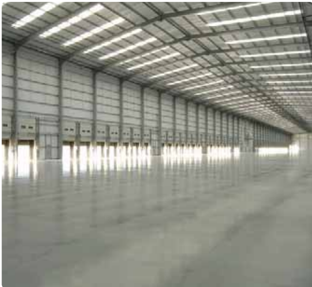
Figure 2: Award-winning completed slab for ProLogis, Peterborough.
