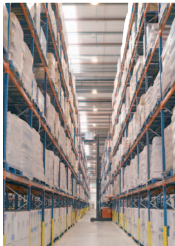
Figure 3: With the correct approach, it is possible to consistently produce very flat floors without the need for remedial grinding.
