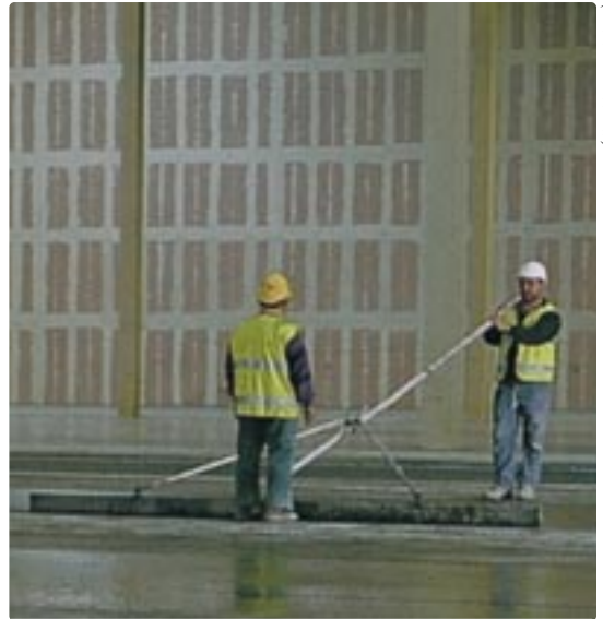
(Photo: Twintec Ltd.)
