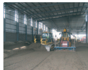
Figure 3: Sub-base preparation using the double-trimming method.
